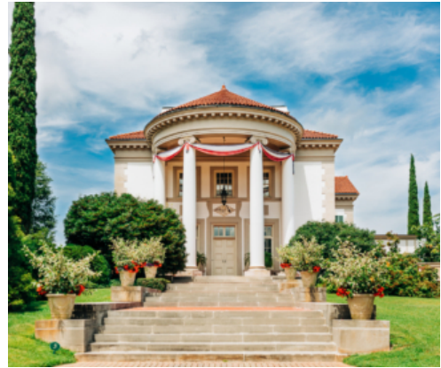
Figure 2- East Portico Entrance
